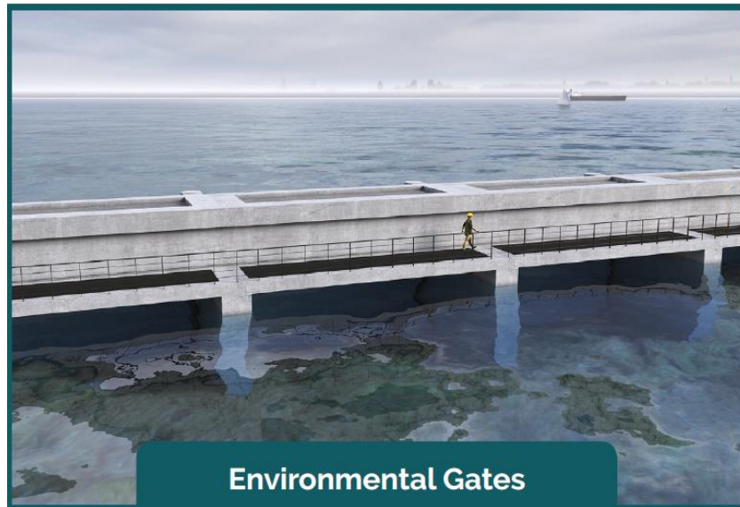
Figure 6-9: Shallow Water Environmental Gates (SWEG) (Conceptual Rendition)
