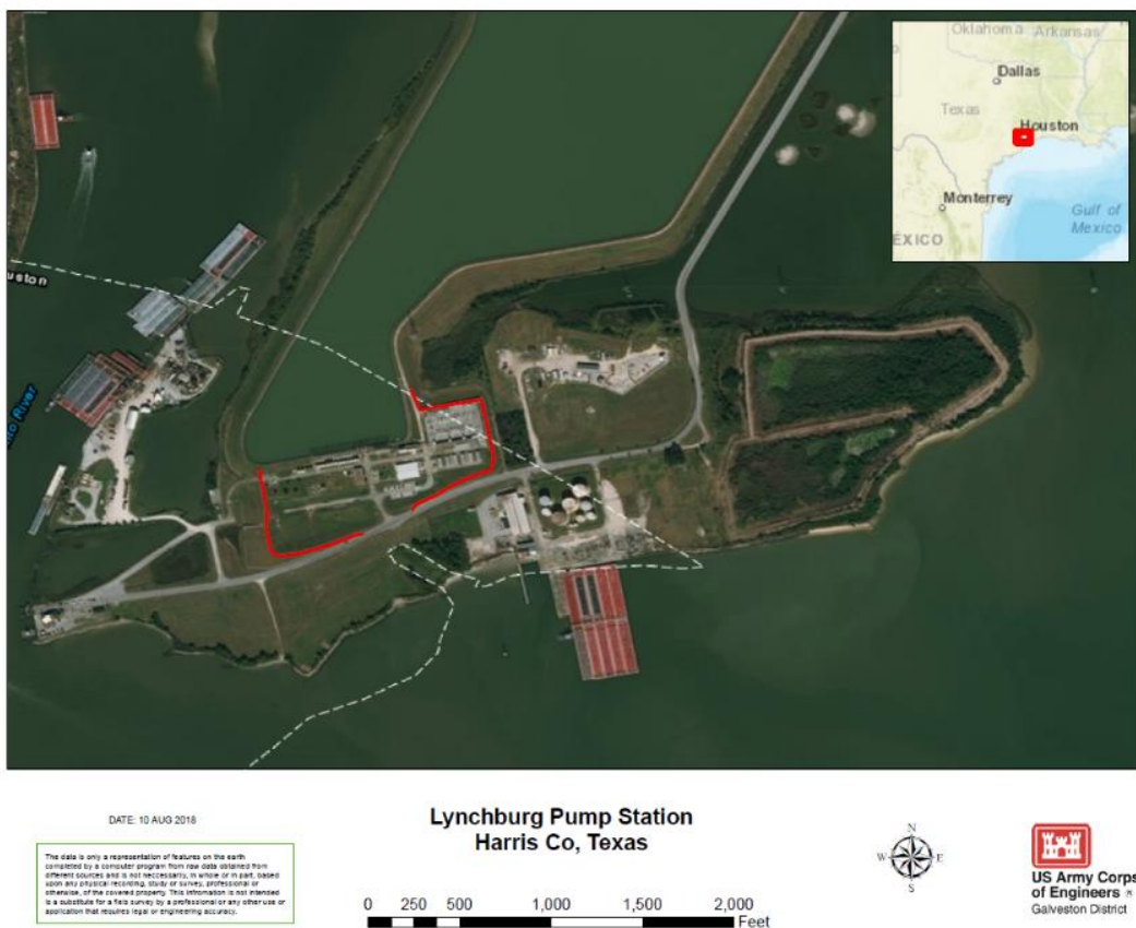
Figure 1-4: Lynchburg Pump Station
